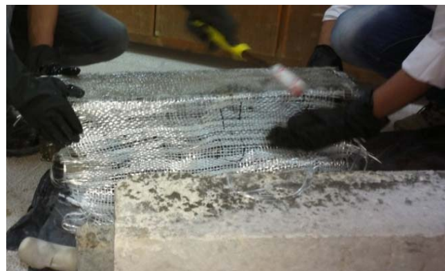
Figure (8) : Installing of Glass Fiber Sheets
