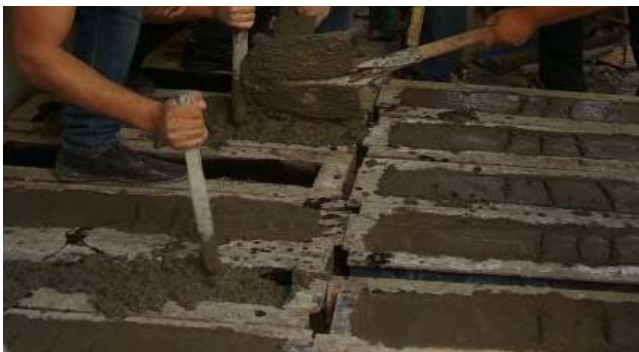
Figure (6) : Compaction Process
