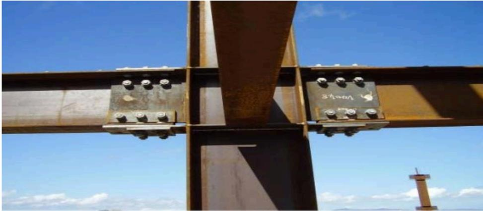
**Figure .2 Sliding Hinge joints**
