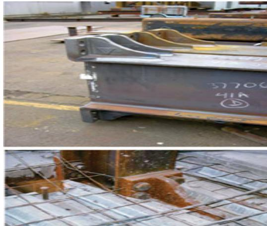
**Figure.10 Kaiser Bolted Bracket Moment Connection**
