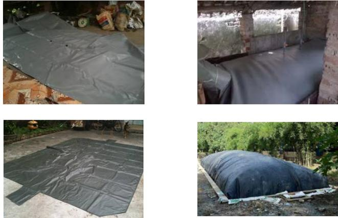
Fig. 2 The plug-flow digester installed in a rural location in Vietnam
