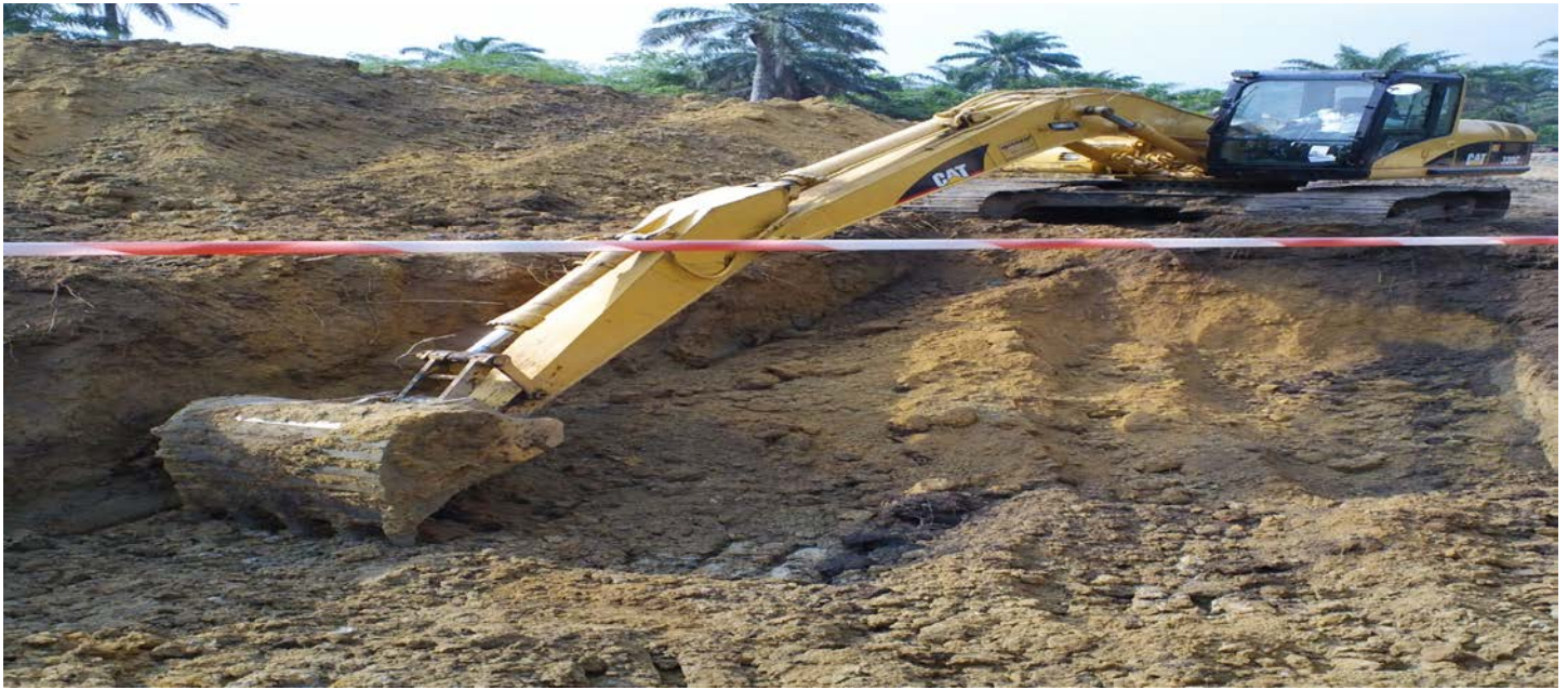
Figure 7.0: Showing excavation of contaminated soil.
