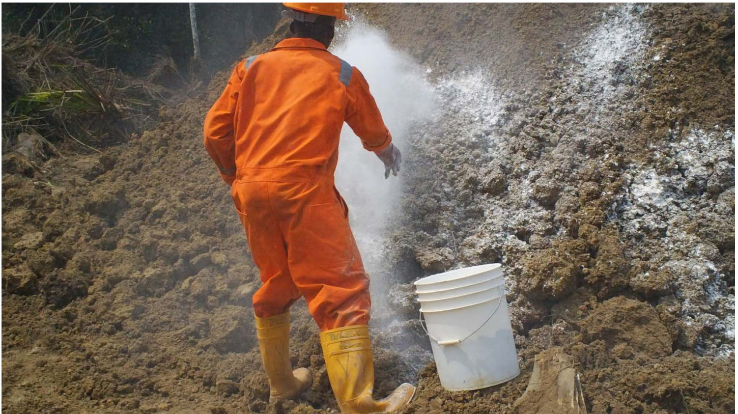
Figure 8.0: Showing hand broadcasting of activated persulfate oxidant.
