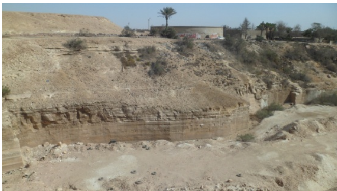
c) Surface water leakage
