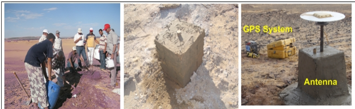
Fig. 3: Construction and Installations of GPS Base Stations
