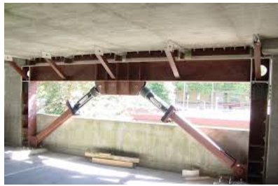
Fig 3 Friction Damper Setup
