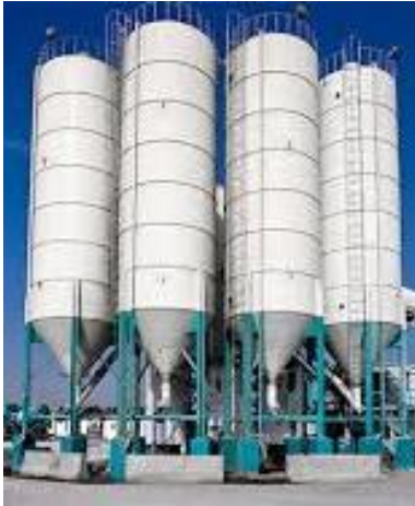
Fig 1 Elevated steel silo
