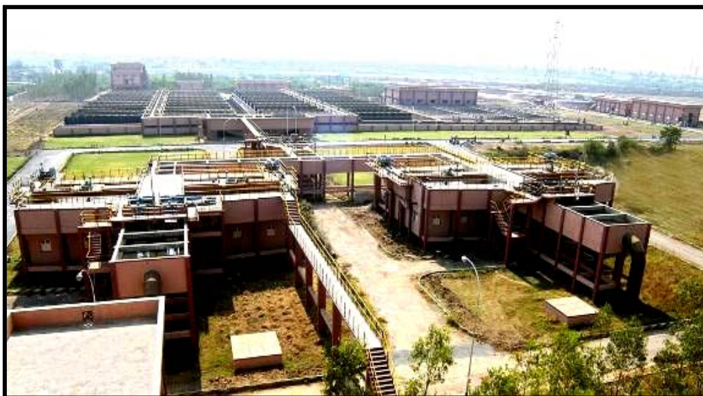
Fig. 2 UASB + EA based 100 MLD capacity STP (phase I), Bamroli
