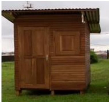
Figure 2: room test on the University of Douala, front view.
