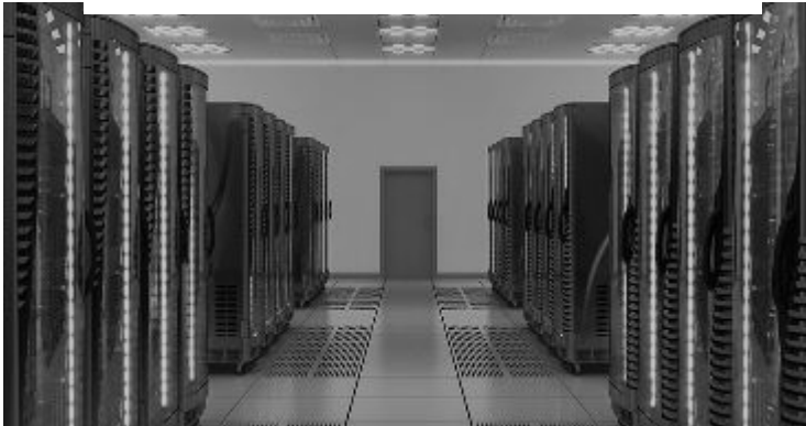
Figure 12: Cloud and Data Warehousing
