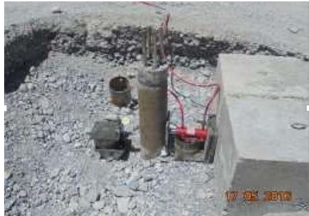
Figure 4: Concrete Testing at Site
