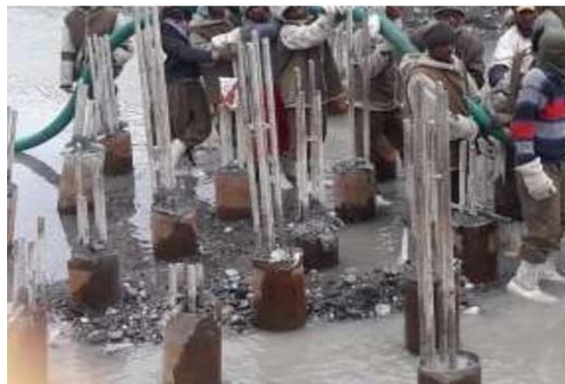
Figure 3: Group Pile Casted with Air Entrained SSC
